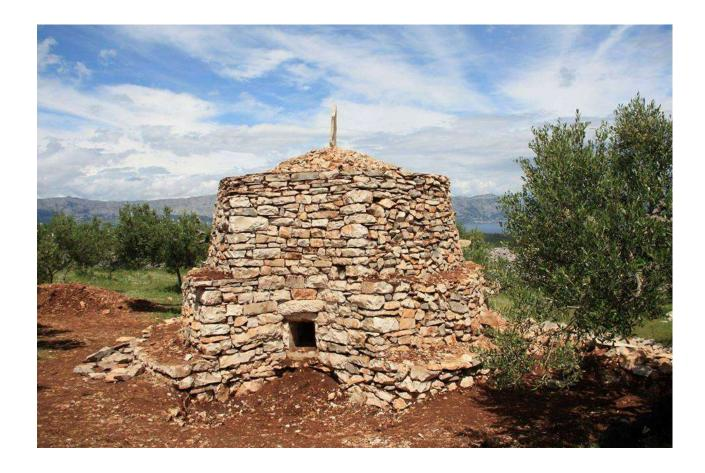
LIMEKILN – "JAPJENICA" – oven for baking lime
